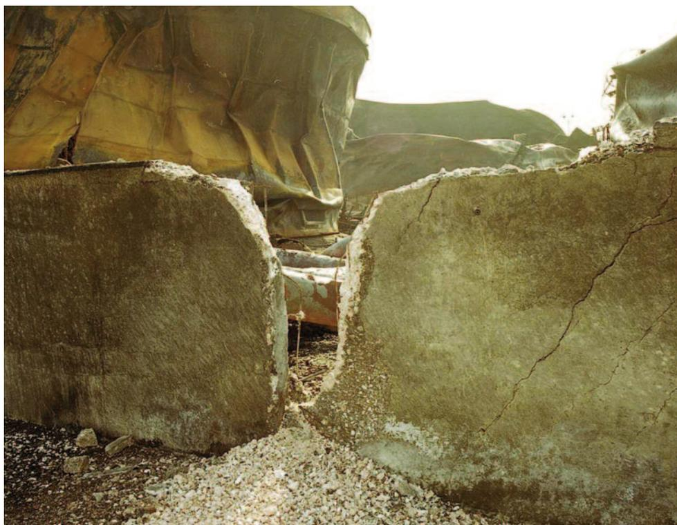
**Figure 8** Failed bunds on the Buncefield site photographed after the fires were all out
