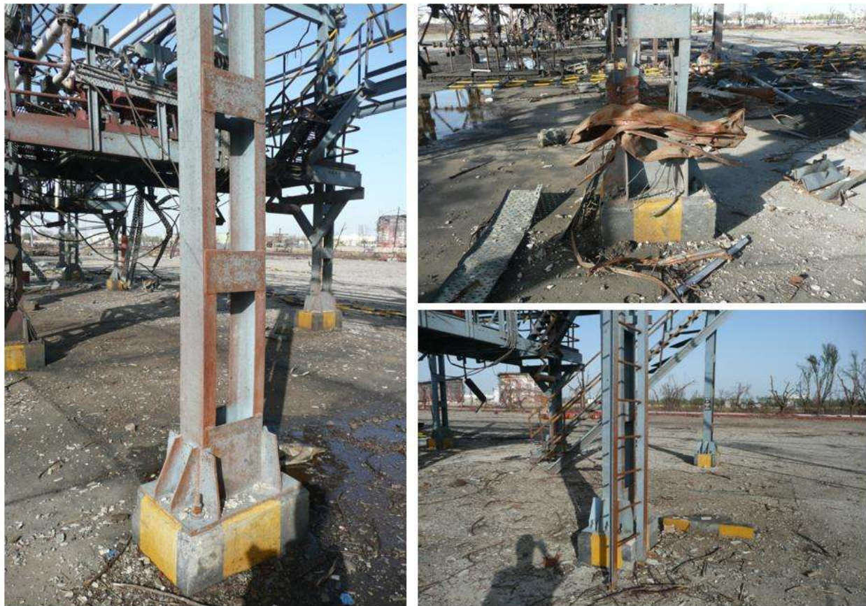
Figure 44: Directional indicators in loading gantry
