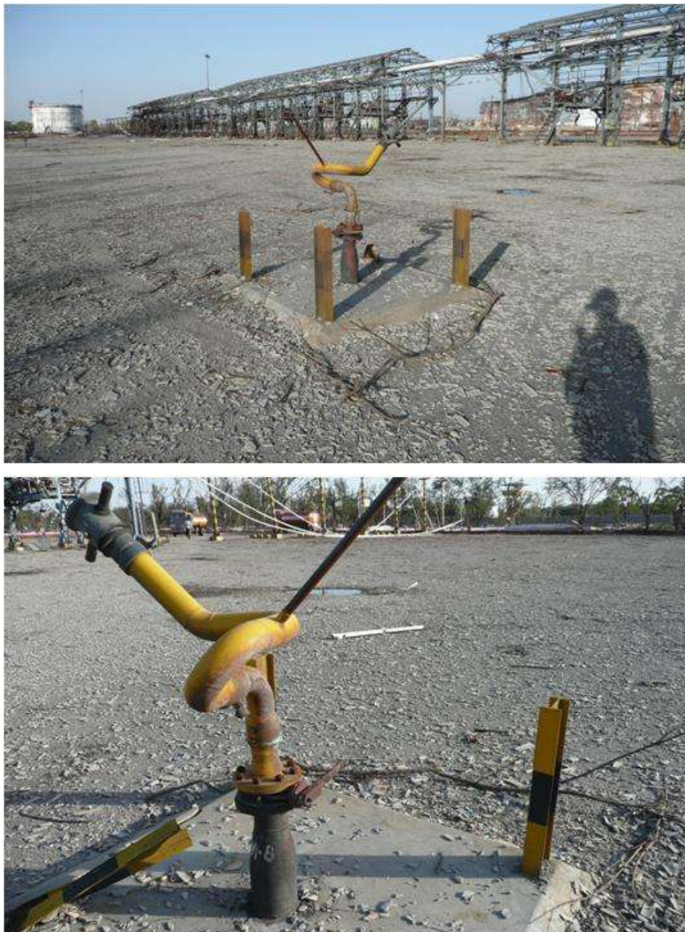
Figure 47: Fire hydrants adjacent to the tanker loading gantries.
