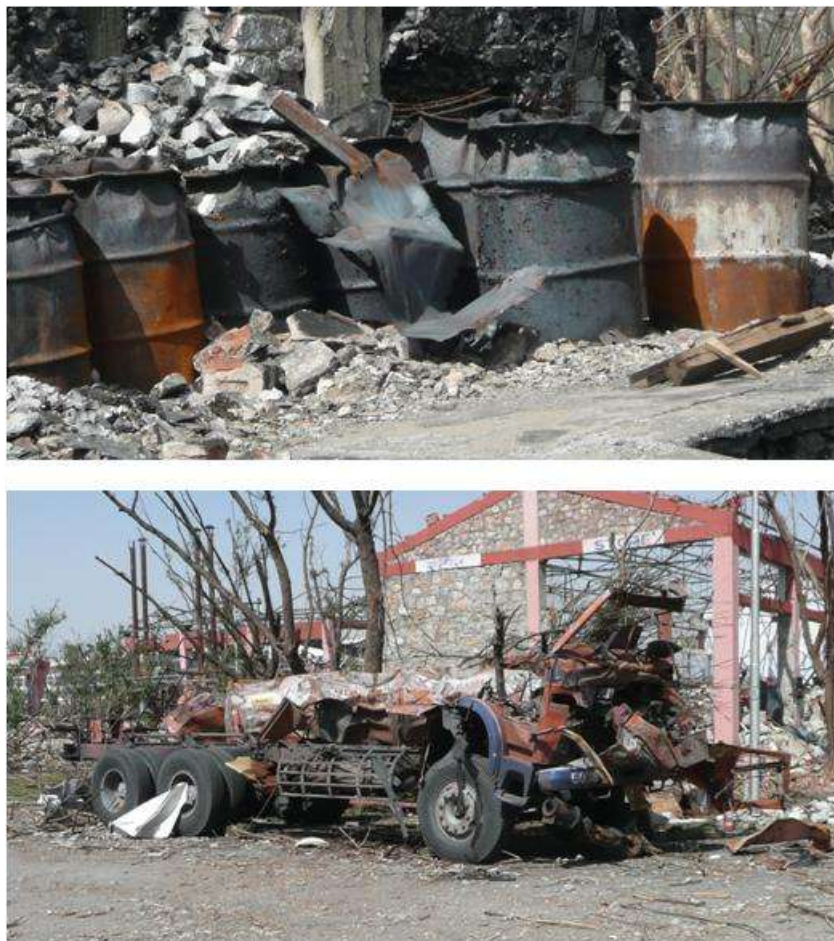
Figure 4: Examples of Overpressure Damage
