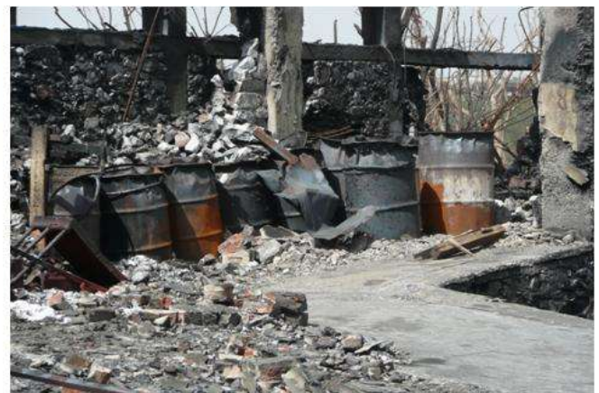
Figure 24: Fire and explosion damage to the warehouse and crushed drums on loading bay
