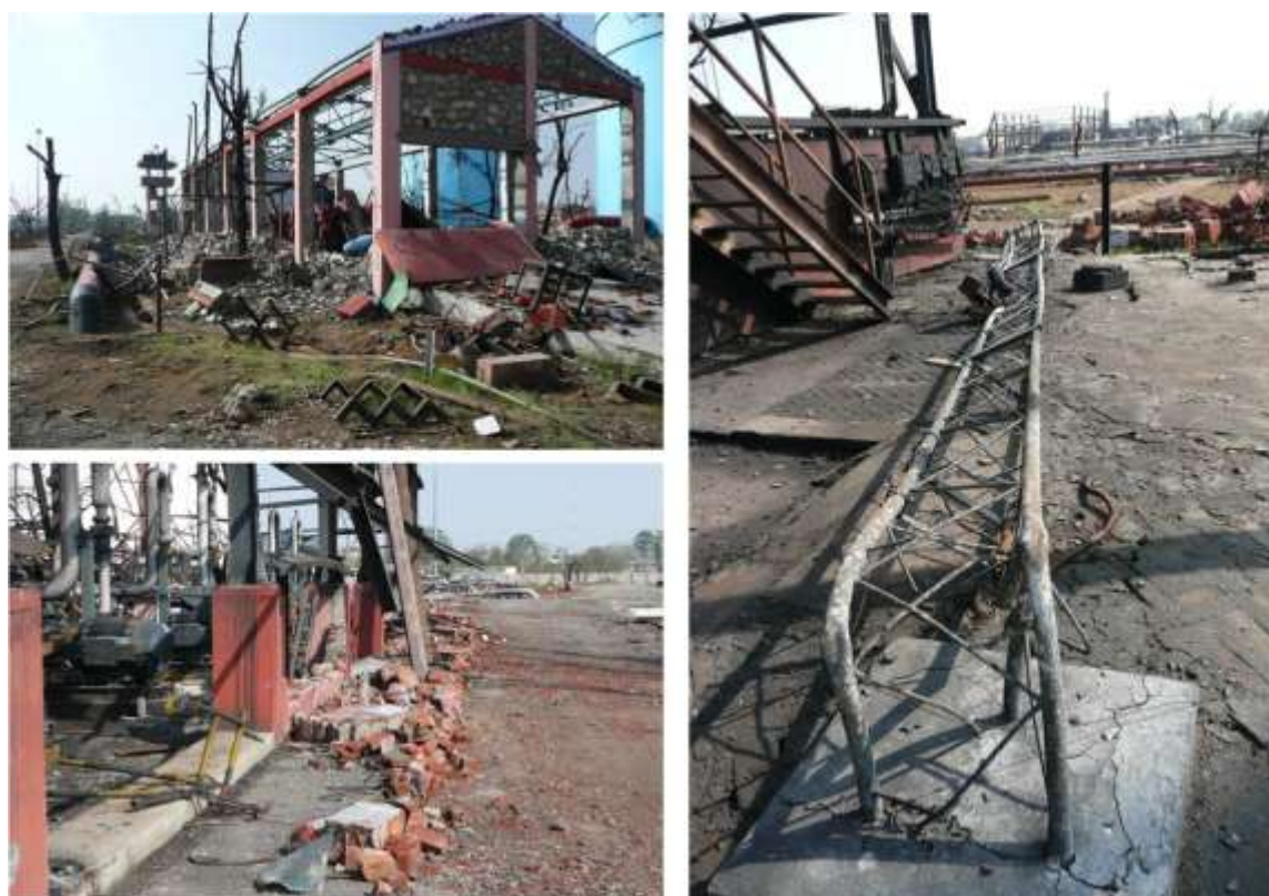
Figure 39: Damage to the firewater building (top left), the main product pump station (bottom left) and a collapsed CCTV tower at the south end of the main product pump station (right)
