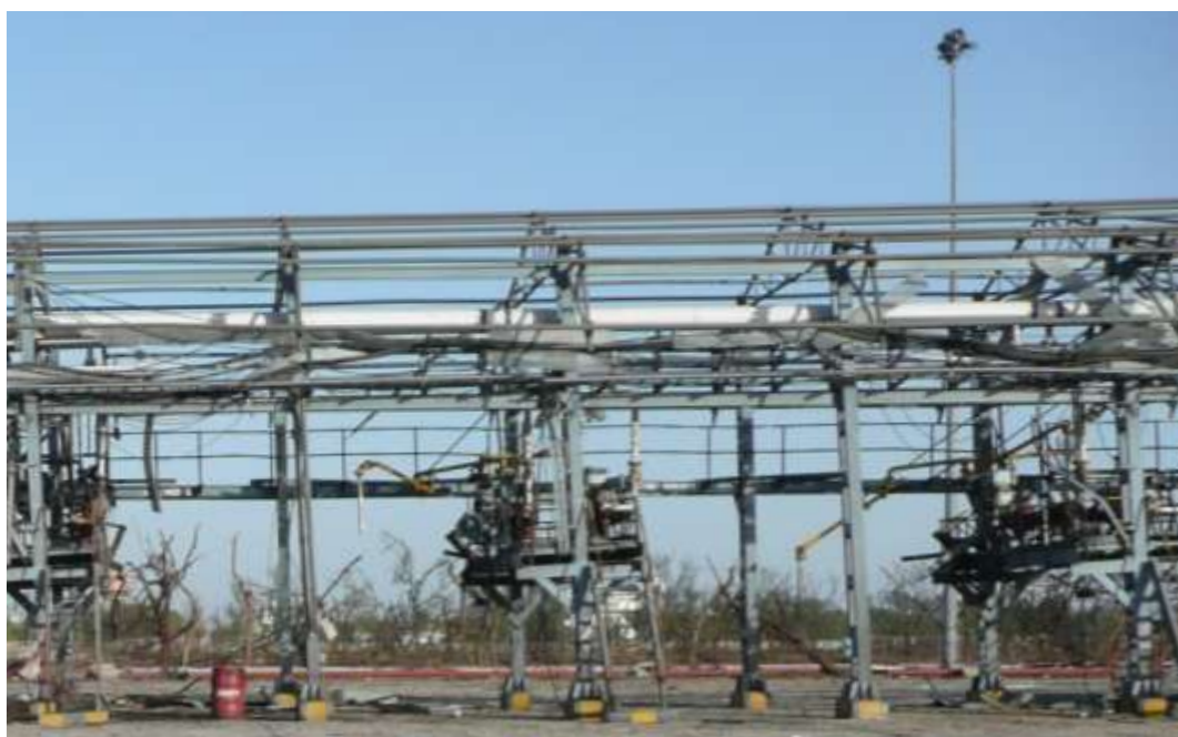
Figure 42: Displacement of the tanker loading gantry (viewed from the west)
