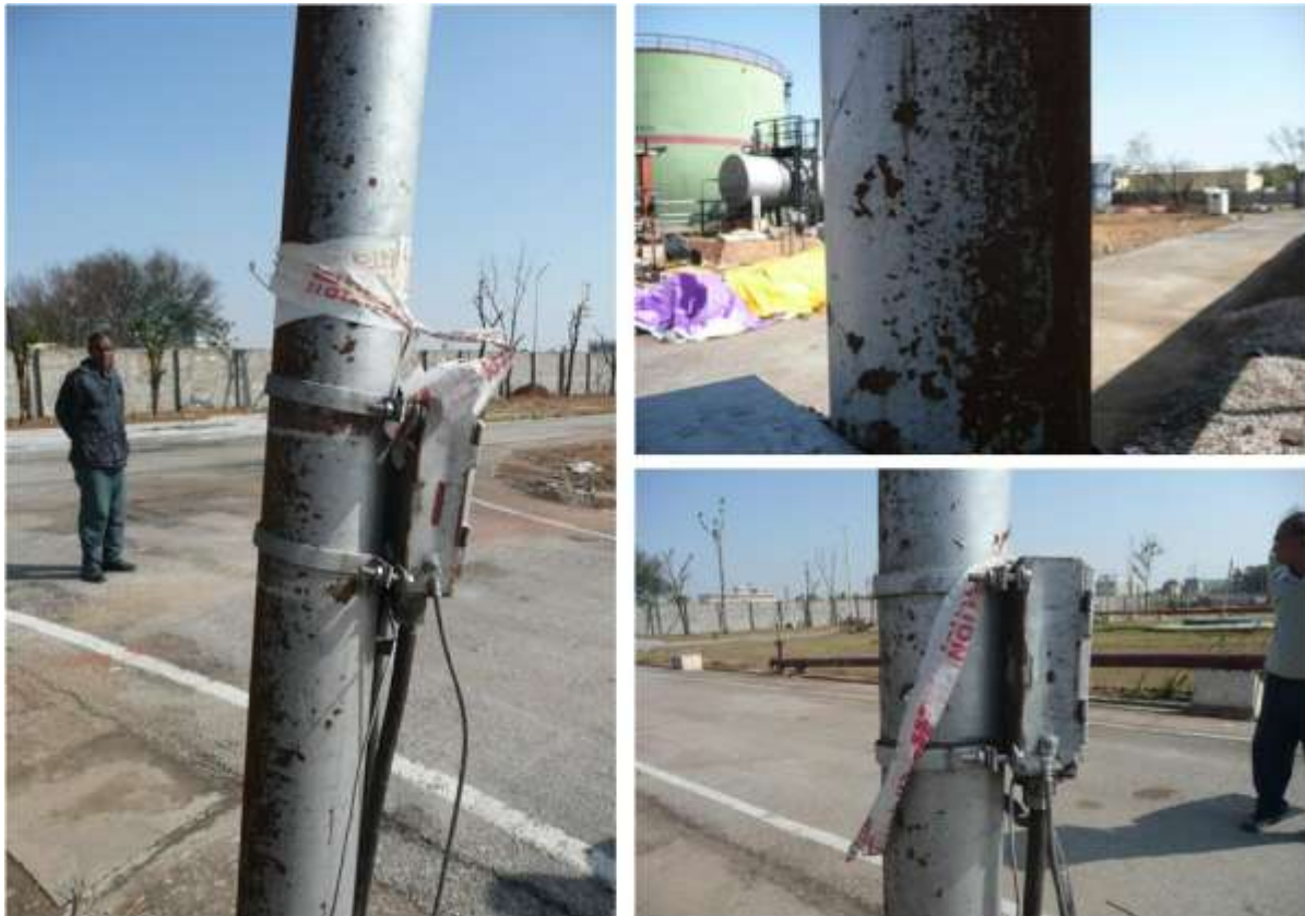
Figure 57: Scouring of paint on lampposts and crushing of boxes
