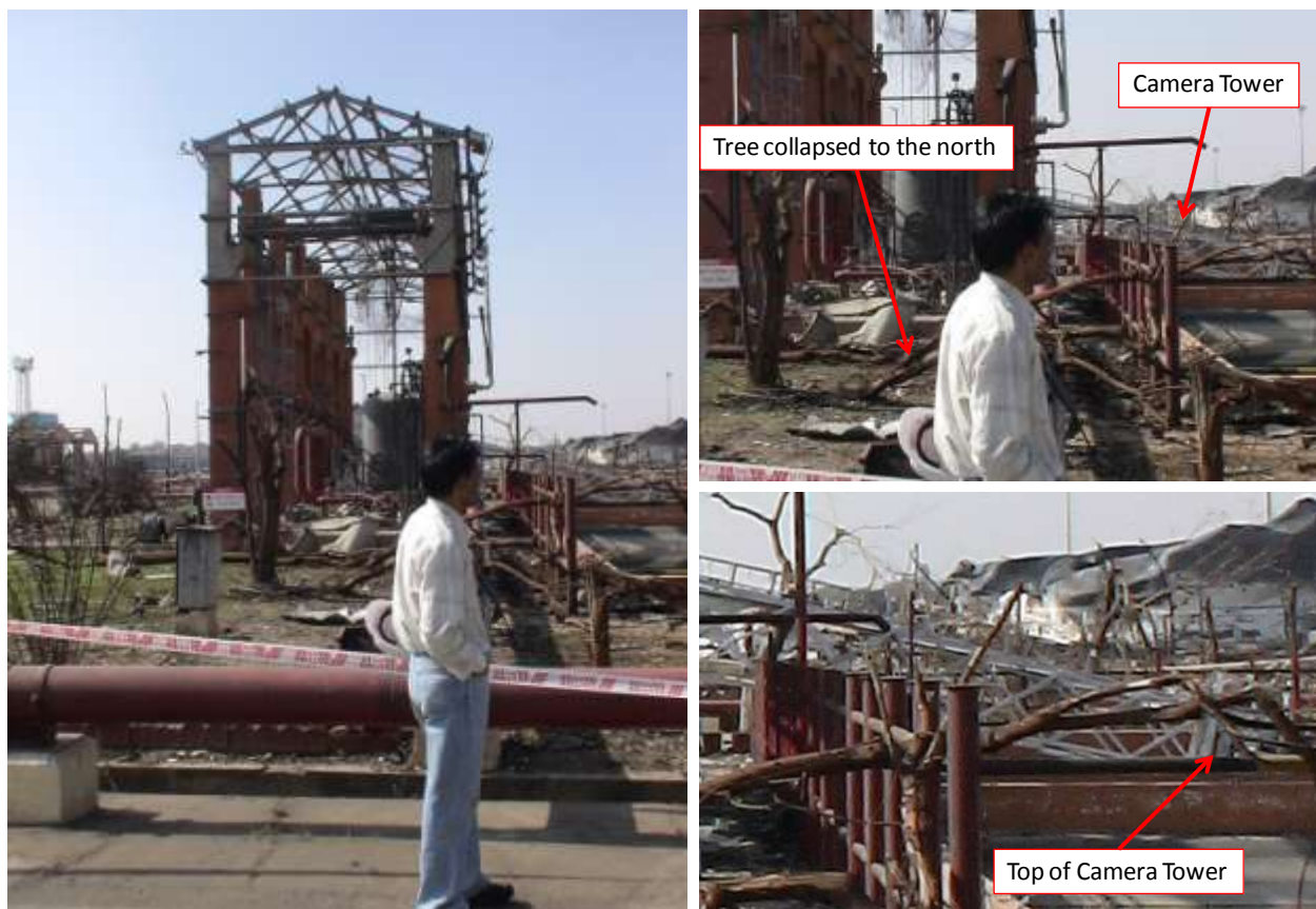
Figure 64: View from the east of the main firewater pump house looking west, showing collapsed trees and camera tower (picture taken by Dr B. Burgan)
