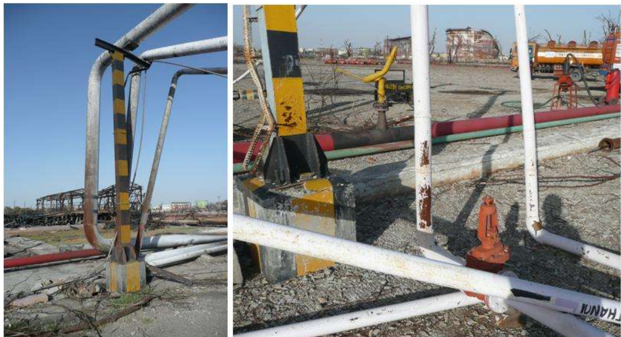
Figure 46: Directional indicators on pipes and supports at the north (left) and south (right) of the tanker loading gantries
