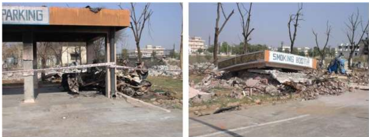
Figure 61: Damaged car in Pipeline Division car park and collapsed smoking booth (pictures taken by Dr B. Burgan)
