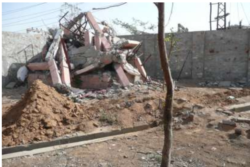
Figure 34: Collapsed guard tower on north wall
