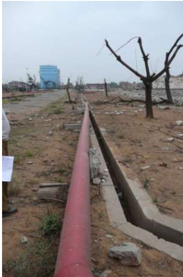
Figure 33: Displacement of firewater pipe to the west
